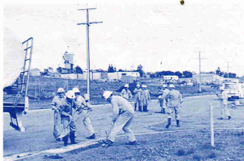
Soil was used to block storm water drain (near opening) to prevent toxic fumes escaping, before being neutralized with water.
